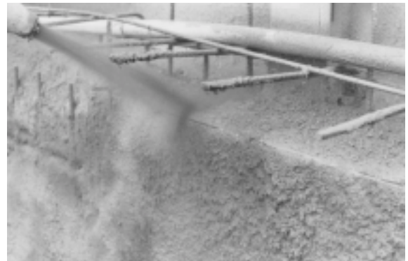
Fig. 5.4—Shooting concrete using ground wires as a guide to bring materials to line and grade.
