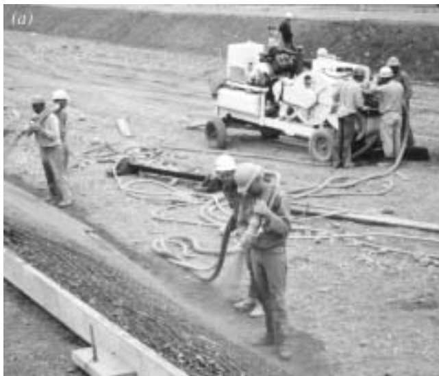
Fig. 1.4—Applying steel fiber-reinforced dry-mix shotcrete against a rock.
