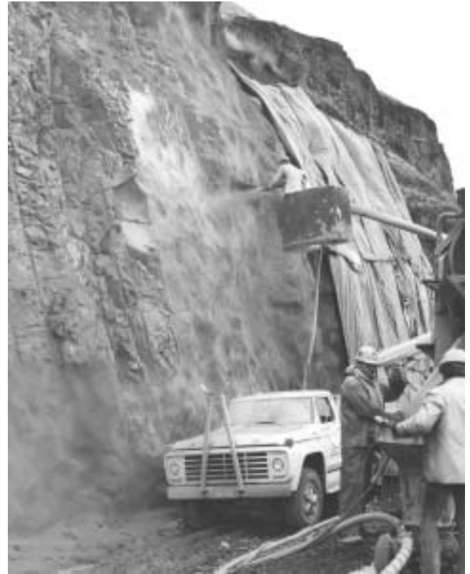
Fig. 1.4—Applying steel fiber-reinforced dry-mix shotcrete against a rock.
