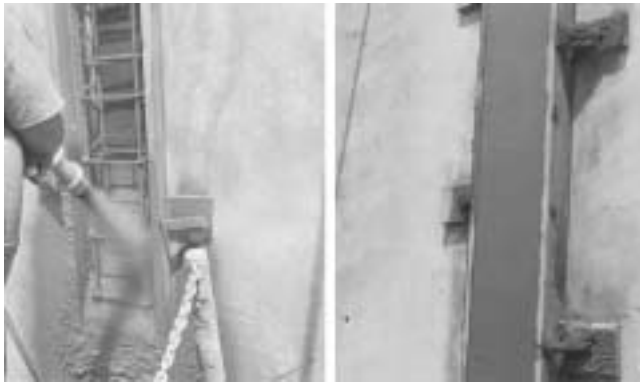
Fig. 8.8—Dry-mix shotcrete pilaster between two concrete tilt-up panels.
