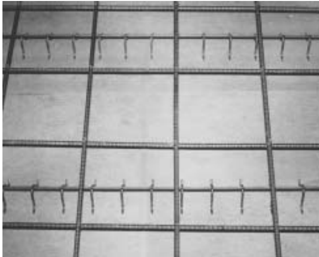
Fig. 5.3—Positioning slab bolsters. Correct (left) and incorrect (right) method for placing continuous chairs or slab bolsters. (To avoid sand pockets, the bolster wire should not be adjacent or parallel to a wire mesh.)
