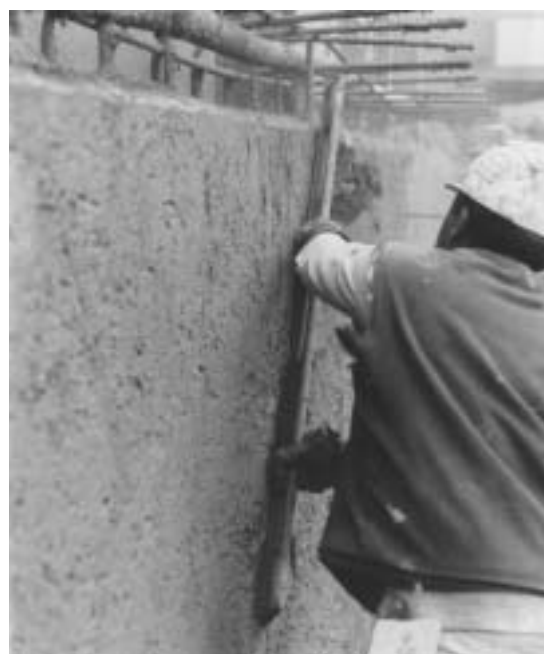
Fig. 8.11—Screeding excess or overgunned shotcrete, leaving a rough, textured finish.
