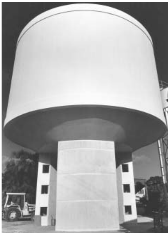
Fig. 1.1—Elevated prestressed shotcrete water storage tank.
