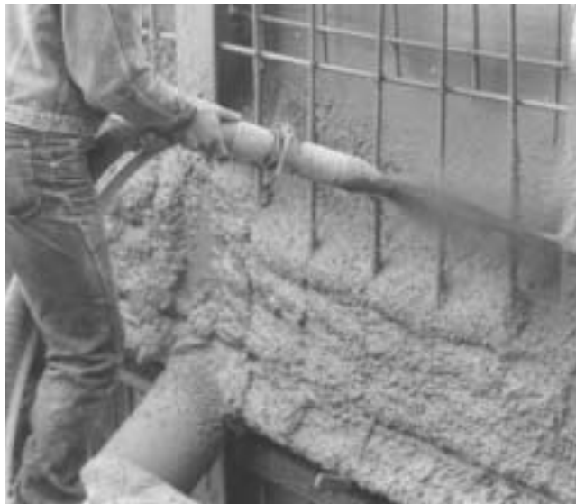
Fig. 8.4—Wet shooting around reinforcing bars.
